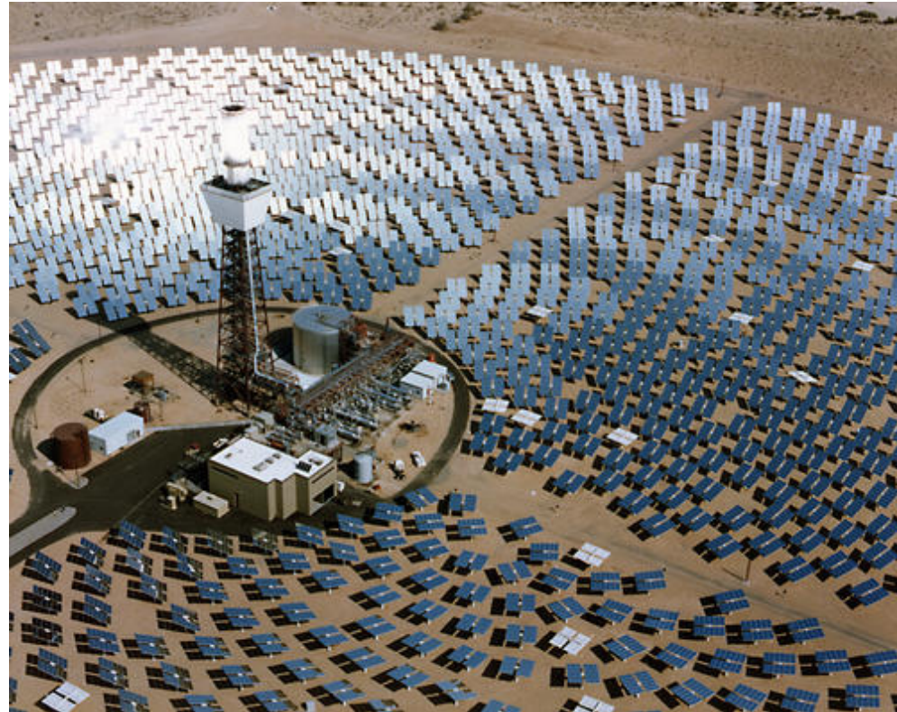
The Solar Two thermal solar power plant. from www.nrel.gov
